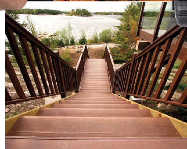
(Above) Bryan and his wife Sarah go over plans for their new family cottage on Georgian Bay that became the focus of the successful "House of Bryan" show on HGTV. The cottage takes shape with snow still on the Bay. Finishing touches include a beautiful staircase down to the water's edge. (Photos courtesy HGTV)
