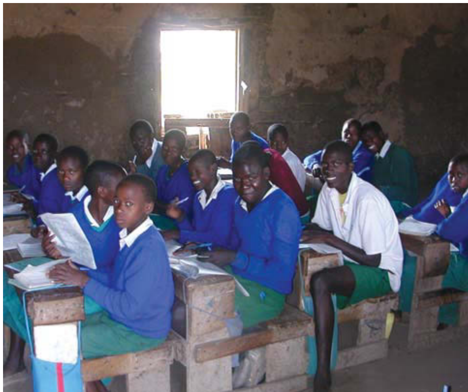
This is an elementary classroom with students from the Mara Region of Kenya. It is an old classroom with dirt floors and walls of mud/dung/sticks with a single window with no glass. Martin Herbst's students worked on construction of a new school to replace classrooms like this. (Photo by Martin Herbst)
