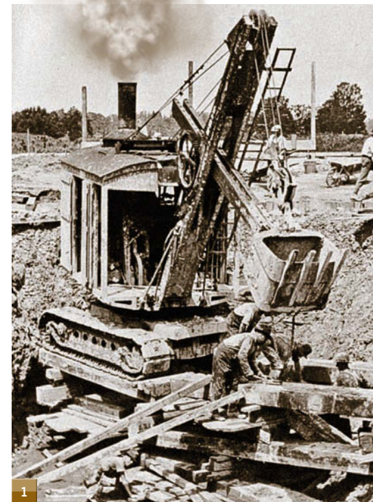
(1) Steam shovel excavating bridge footings, 1922. (2) 'Teamsters' haul sand and gravel. Contractor John Putherbough is seen standing in the foreground, white shirt, hands behind his back. (3) University Bridge circa 1935. (4) First and last house over the bridge, 1955. (5) Cement mixer used in bridge construction in 1922.
