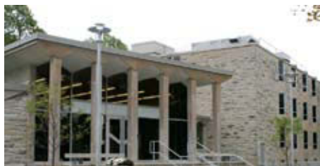
Newly renovated Westminster College.
